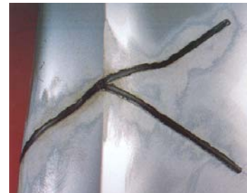
Completed Weld ready for finishing and painting
